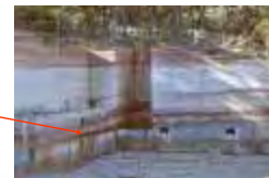
Groundwater seepage from bedding plane in sandstone
